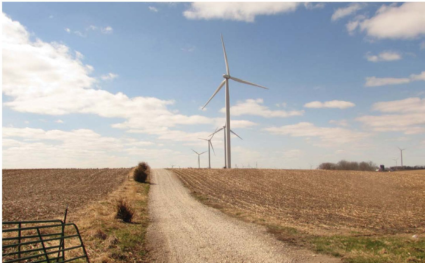
Photographer: Parker Taylor | Windmill construction attracted workers to our region and brought resources to our high school for much needed improvements.
